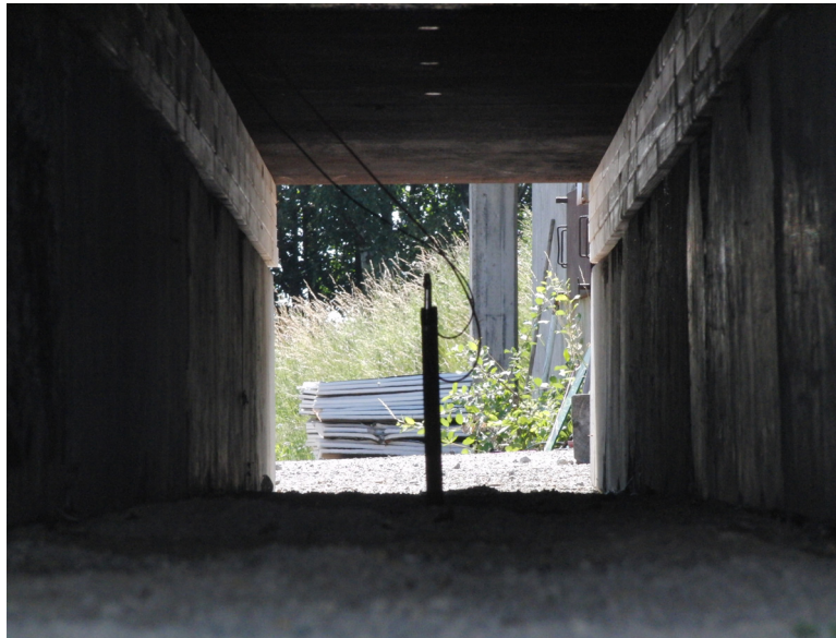
Figure 8. Inside tunnel view
