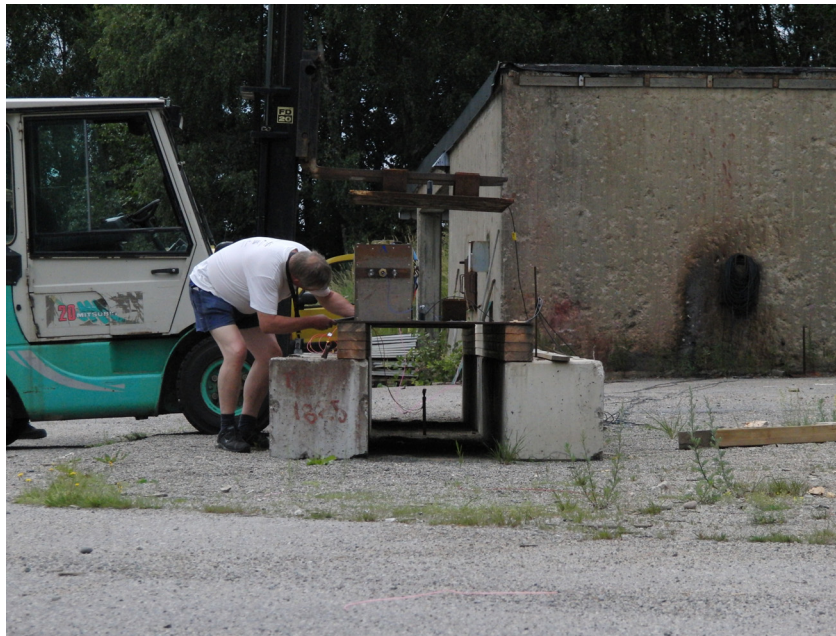
Figure 12. Camera view of tunnel
