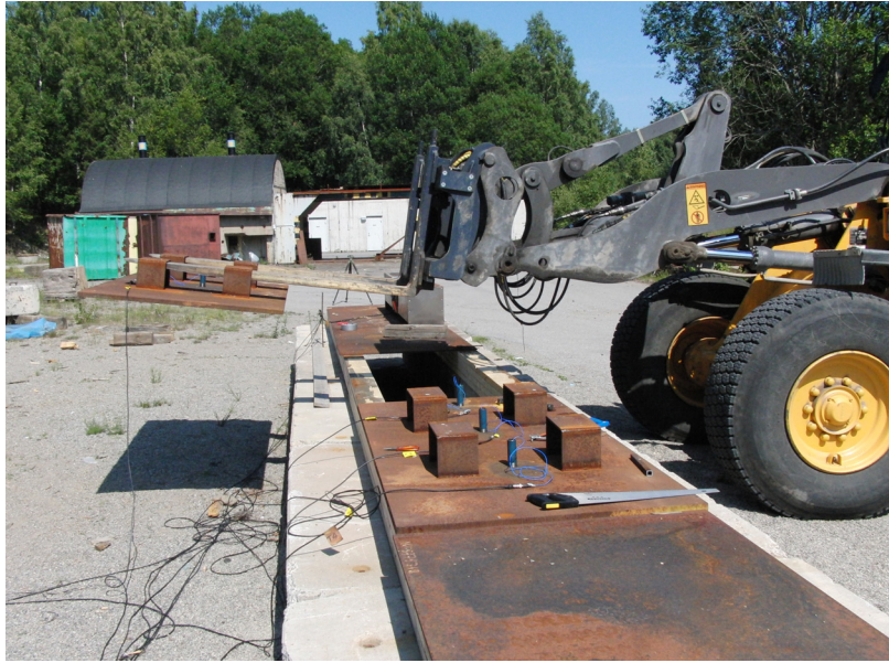
Figure 9. Outside tunnel view
